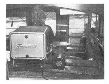
Left - Radio equipment and power - supply unit on the Diesel locomotive No. 900
